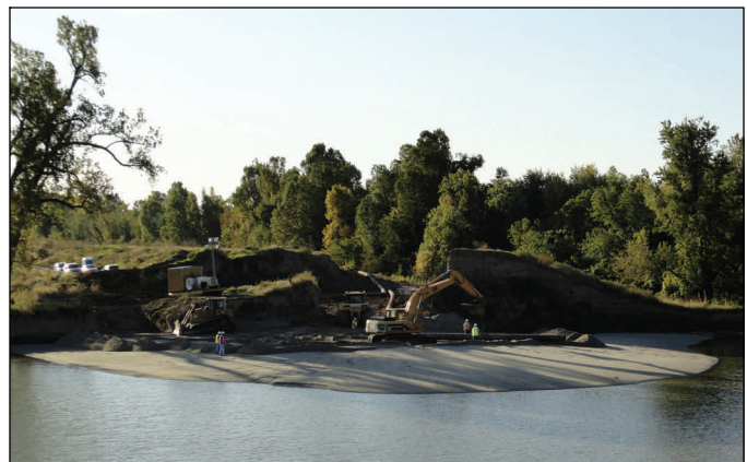
The dredge contractor adds discharge pipe Friday to continue pumping sand into the center crevasse.
