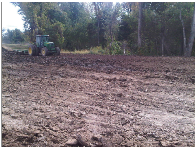
A Vicksburg-based operator prepares a 300-foot-long washout for repair near the lower crevasse Wednesday.
