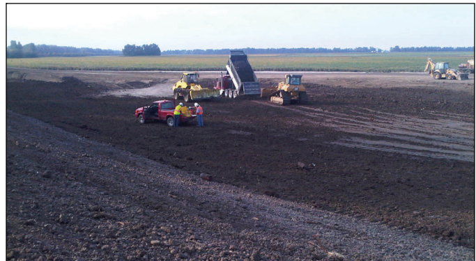
Clay embankment is placed in the final scour hole at the upper crevasse Wednesday to prevent seepage.
